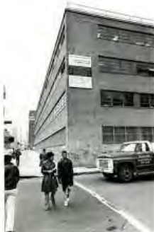
Old North Hall Building
